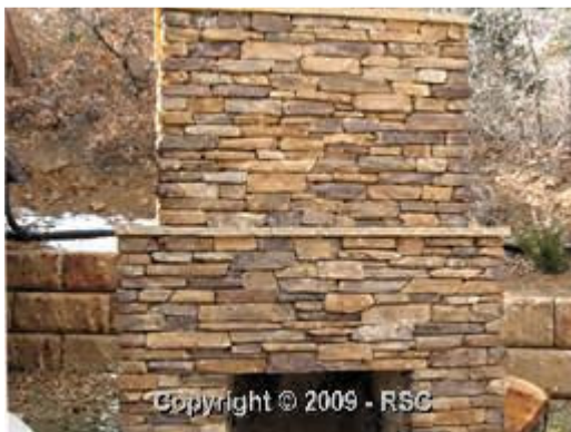
18 x 16 partially covered, stamped concrete patio with handsome 3-tier outside stone fireplace.
