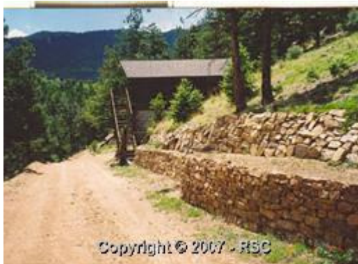
Far off shot of the garage.
